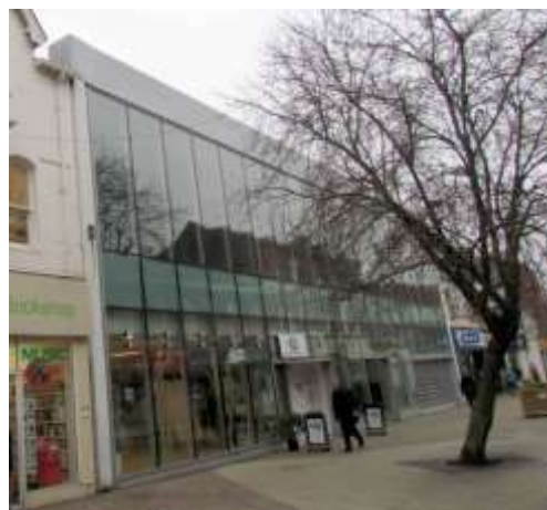
Nos. 74-84 George Street, incongruous for its design as well as its scale and massing
