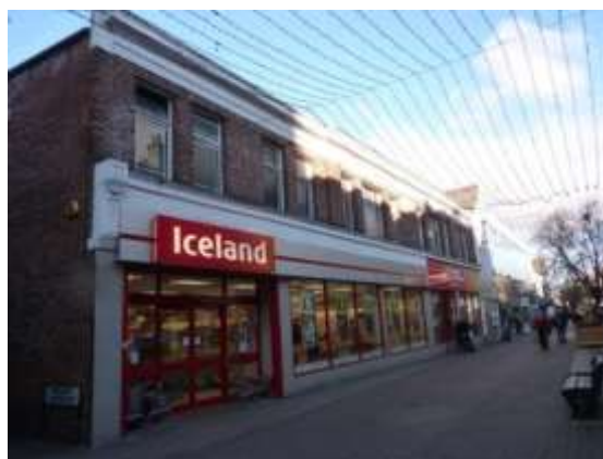
Nos. 88-90 George Street, which has a surviving historic corbel and classical parapet cornice
