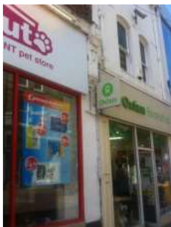
A corbelled fascia end
