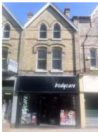
No. 99 George Street, with its original windows
