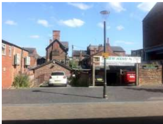
Attractive rear elevations unhindered by inappropriate modern development at the north end of Central Way but with potential for further enhancement through improved boundary treatments and re-location of intrusive features such as the air-conditioning units
